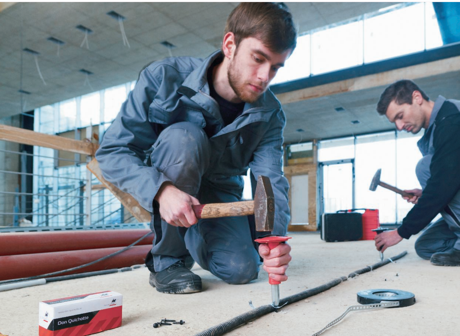
Fastening and supporting, e.g. with fixpin, setting tool and mounting strip
